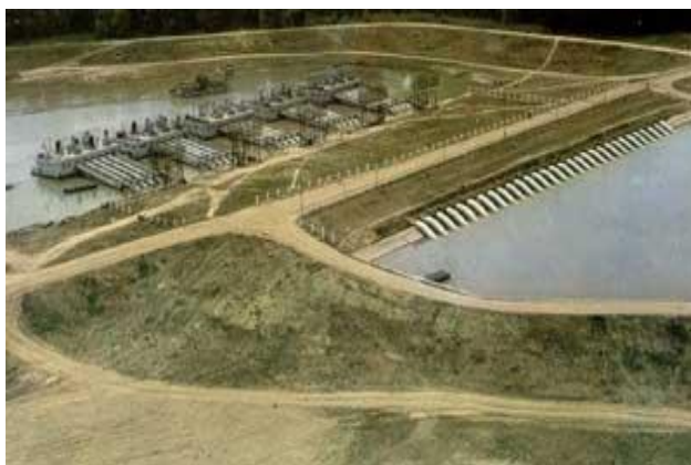
Photo 1. Floating pump station - Irrigation system Gălățui-Călărași
