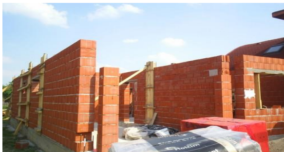
Fig. 2. Structure of Porotherm ceramic blocks Source: www.constructii-neamt.ro [11]
