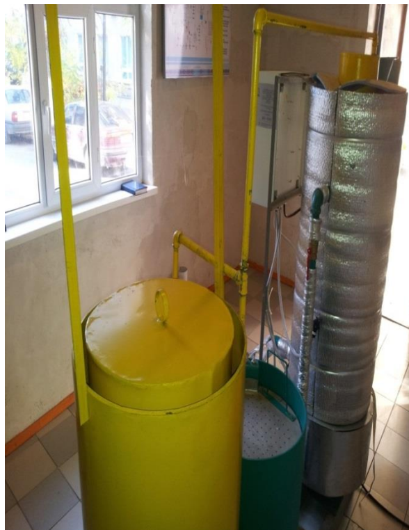
Photo 1. Experimental setup for the biogas production List 1
