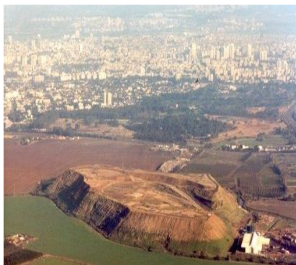
Fig. 1. Storage cell in an ecologic landfill near a city Source: www.greenprophet.com
