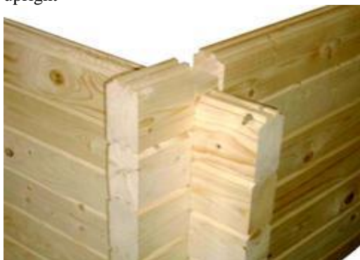
Fig. 3. System with overlapping beams - without interior upright
