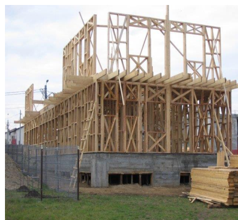
Fig. 2. Foundation and structure of ecological wooden houses
