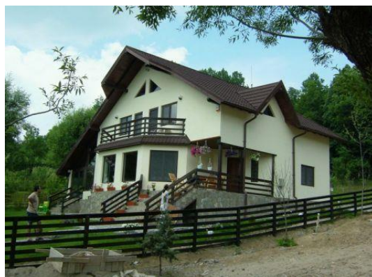
Fig. 3. Ecological house built in Wood Framing System
