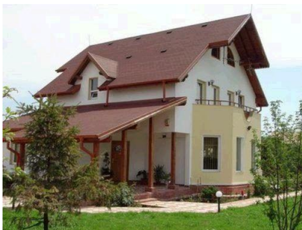
Fig. 4. Ecological house built in Wood Framing System
