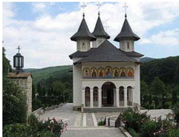
Photo 2: Sihăstria Monastery – Neamţ County
