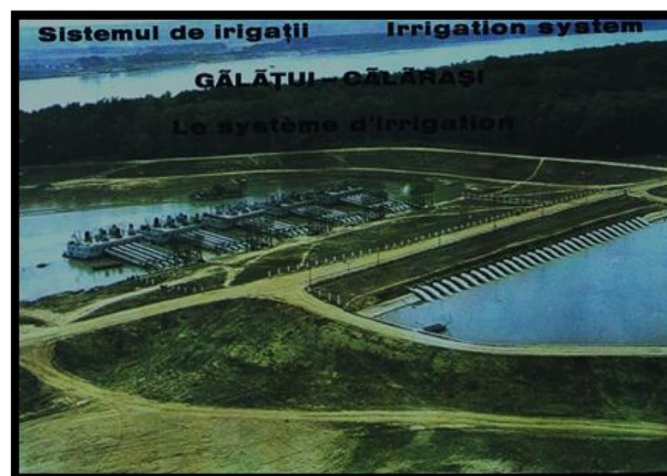
Fig.5. The floating pumping station of the irrigation system of GALATUI, Calarasi County
