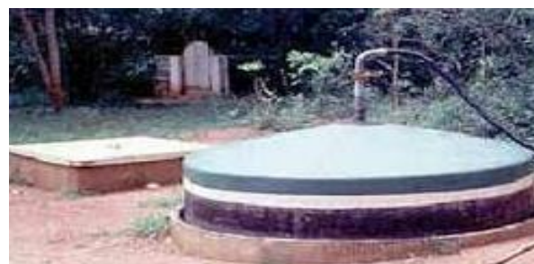
Photo 2. Floating dome or Indian Biodigester fully operational.(Taken fromASOBIOGAS.com).
