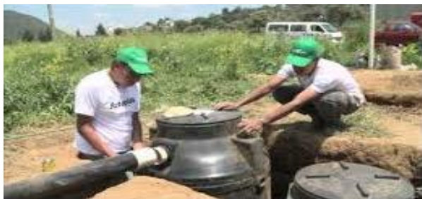
Photo 1. Installing biodigester septic tank.(Taken from Eternit.com)
