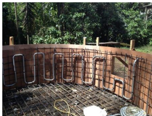
Photo 9. Internal cooling system of the digester. (Taken from Carlos Saborio's investigation).
