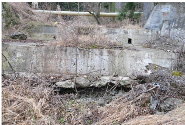
Fig. 3. Undermining of the body of a work
