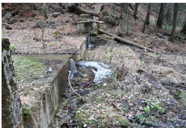
Fig. 4. Dam with clogging in spillway and in apron
