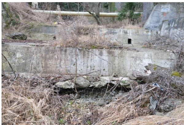
Fig. 3. Undermining of the body of a work
