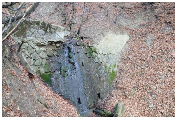
Fig. 2. Damages located to the side of the spillway
