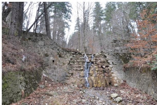
Fig. 1. Dam with damages in the overflowed area
