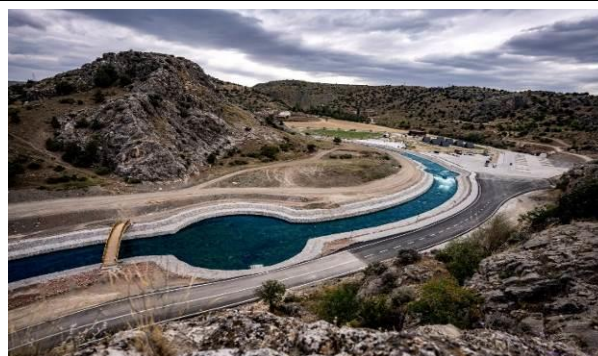
Photo 1. Rafting Area (Çekerek district) Source: [12].
