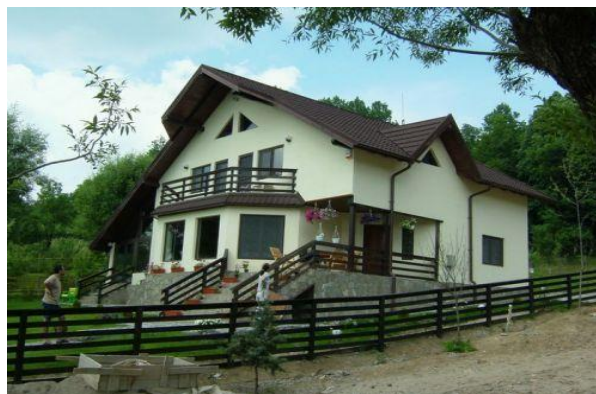
Fig. 3. Ecological house built in Wood Framing System
