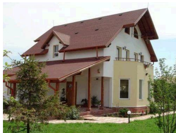
Fig. 4. Ecological house built in Wood Framing System
