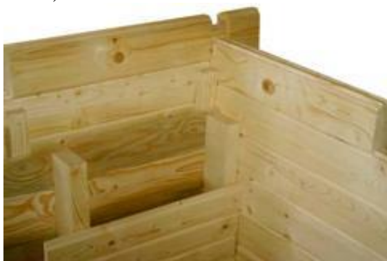
Fig. 2. System with overlapping beams - the interior upright
