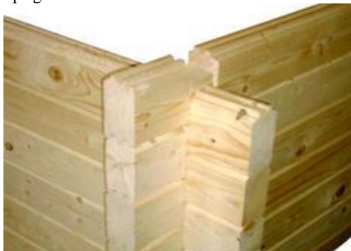
Fig. 3. System with overlapping beams - without interior upright
